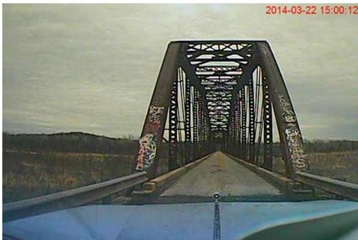
Canadian River Bridge
